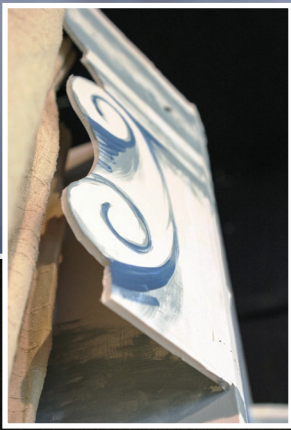
◀ A close-up of the crown molding detail made of inexpensive foam core—available at any arts & crafts store.
